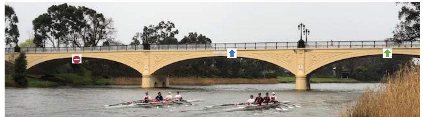
Morell Bridge - travelling upstream
