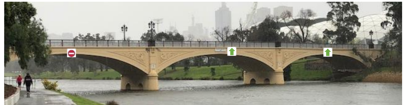
Morell Bridge - travelling downstream
