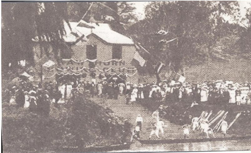
HRC clubhouse built in 1887 north of Bridge Rd—damaged by fire in 1923
