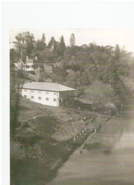
Landing under construction in early 1950's. Xavier was not on site until 1957
